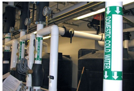
Rainwater cisterns in the basement. Photo: Better Buildings for Oregon
